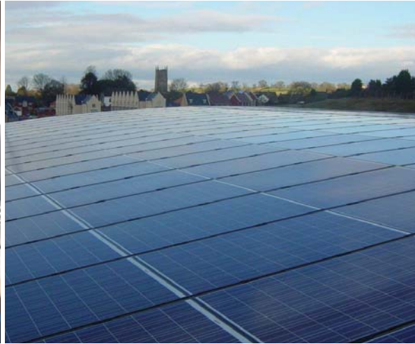
Our 50kW solar array on the Everhot Assembly Plant
